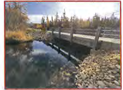
East Main Street Bridge - Manton, MI
